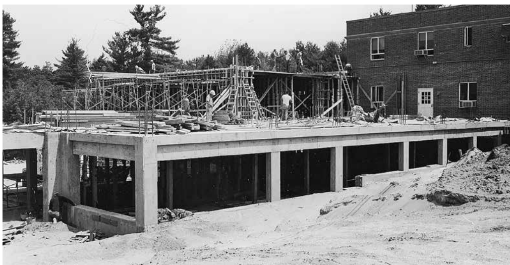
Construction of the new wing, 1965.
