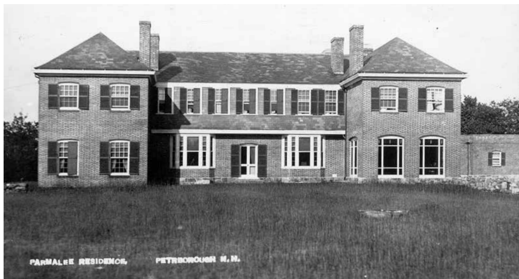
The completed Parmelee House situated on a hill amid the quiet pine woods, with outlook to Mount Monadnock on the west and the lesser, or Pack Monadnock to the East.
