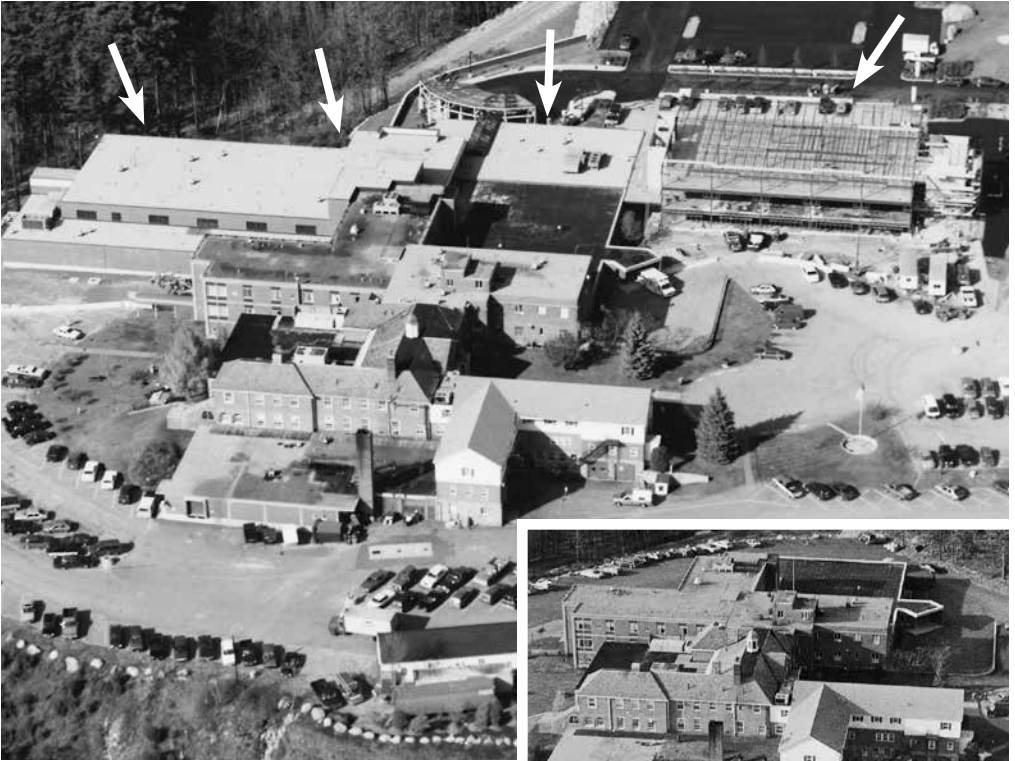
Arrows point to new addition (above). Preconstruction view of the Hospital (right).
