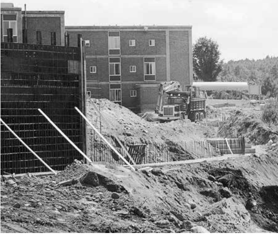
Construction of the 1991 addition.
